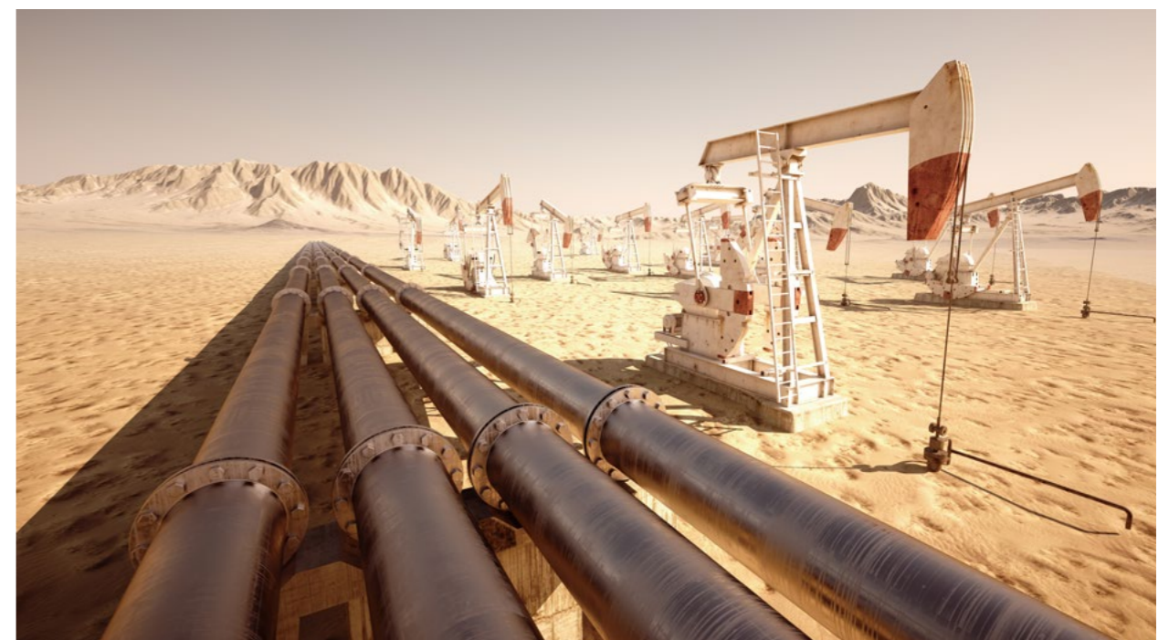
Oil field pipeline
