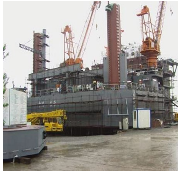
Acid Gas Exhaust System of Drilling Unit Platform
