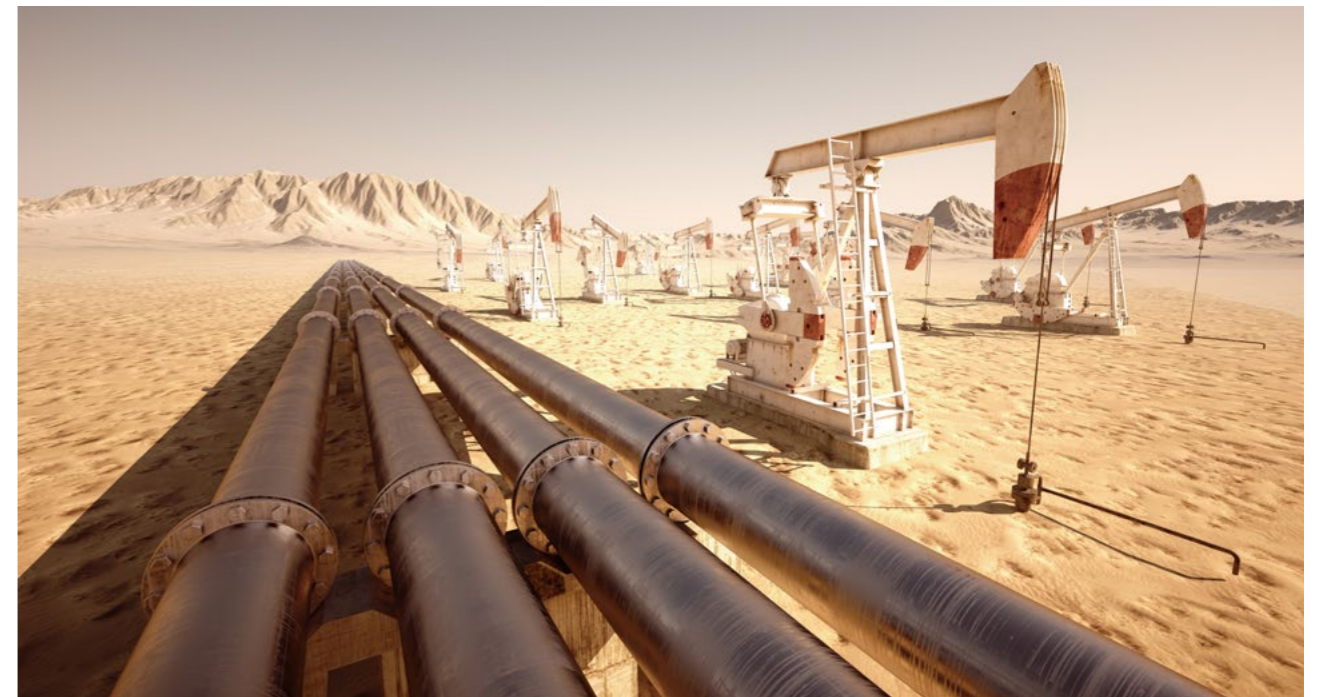
油田管路 Oil field pipeline
