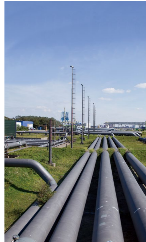
化工厂 Chemical plant
